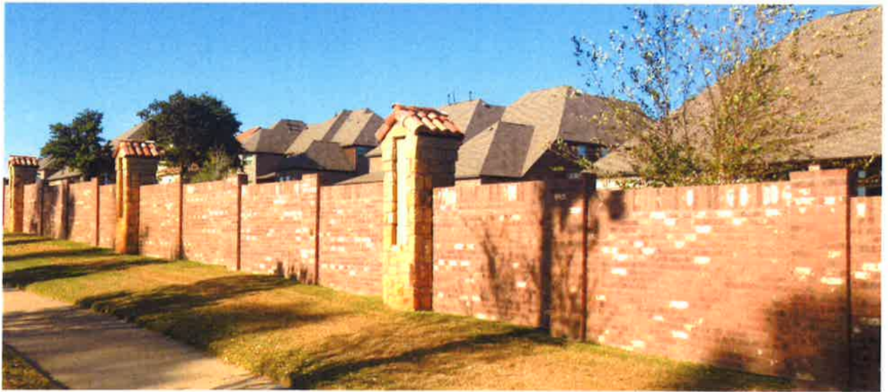
Example of Masonry Screening Wall
