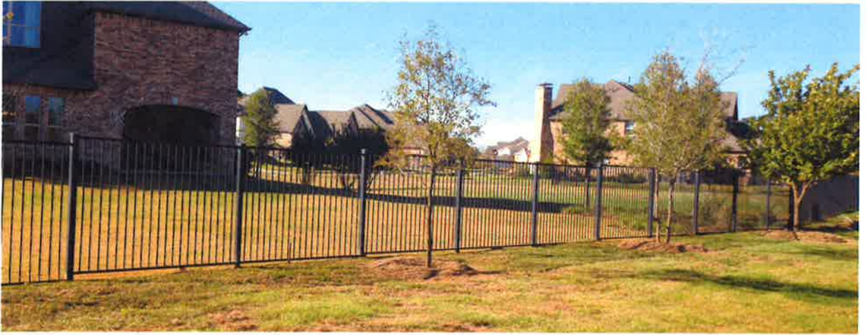
Example of Wrought Iron Fence Adjacent to Open Space
